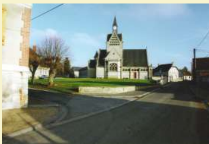
Le village reconstruit de Nanteuil-la-Fosse
