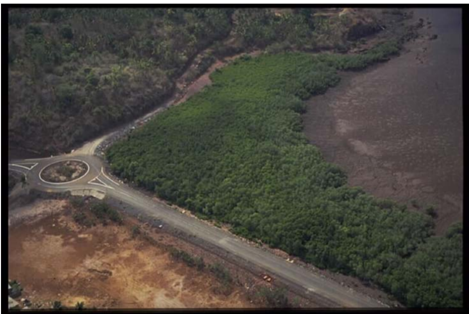
Remblai mangrove Mgombani
