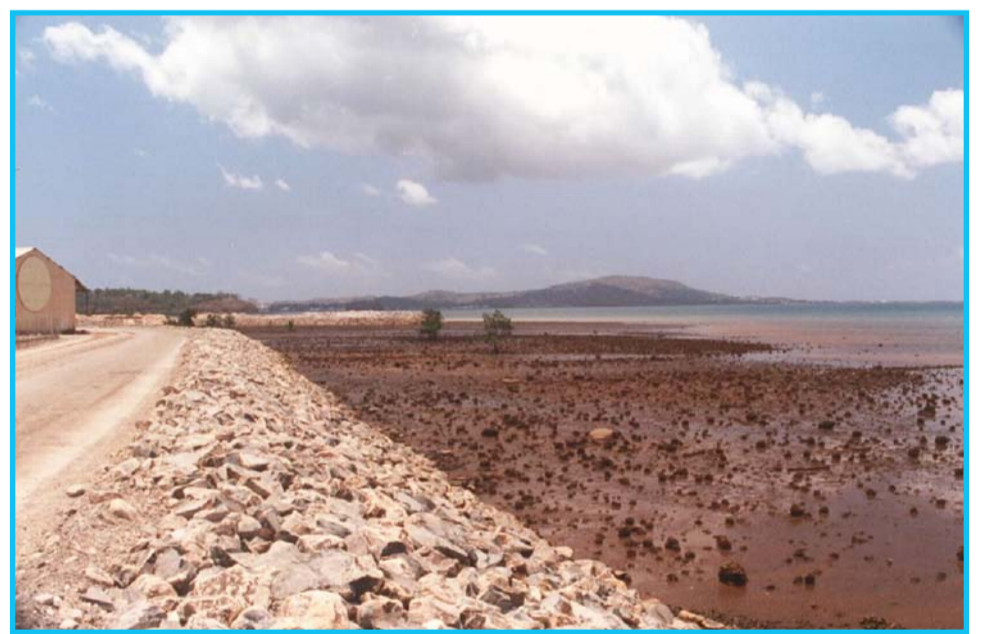
Remblai mangrove Mtsapéré
